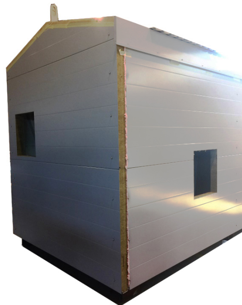
A view of the under-construction instrument container.
